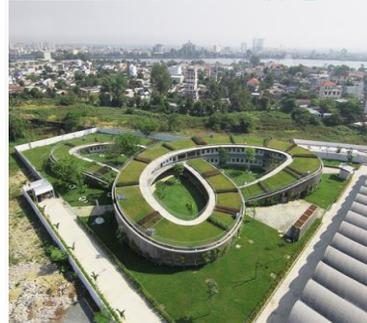
The ingenious shape makes an unusual building, but also maximises airflow around the school, meaning it needs no air conditioning. It is solar powered. That building on the right is a shoe factory whose big roof collects rainwater for the school.
